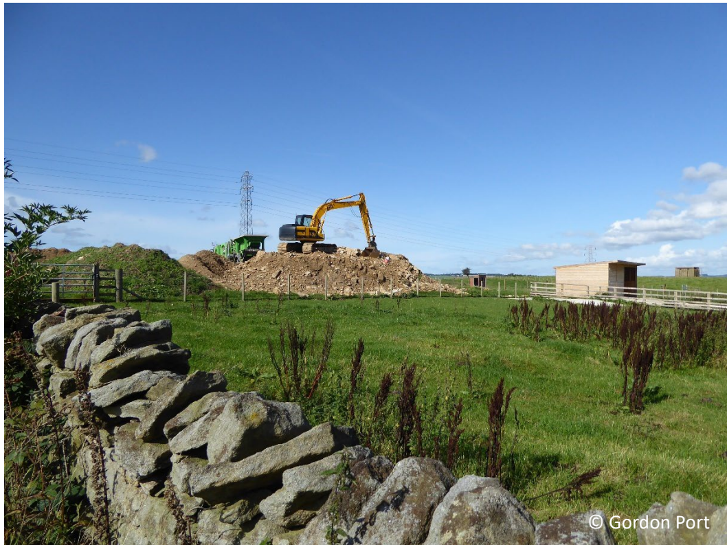
P4 Looking west earthworks near Pasture House farm. September 2023
