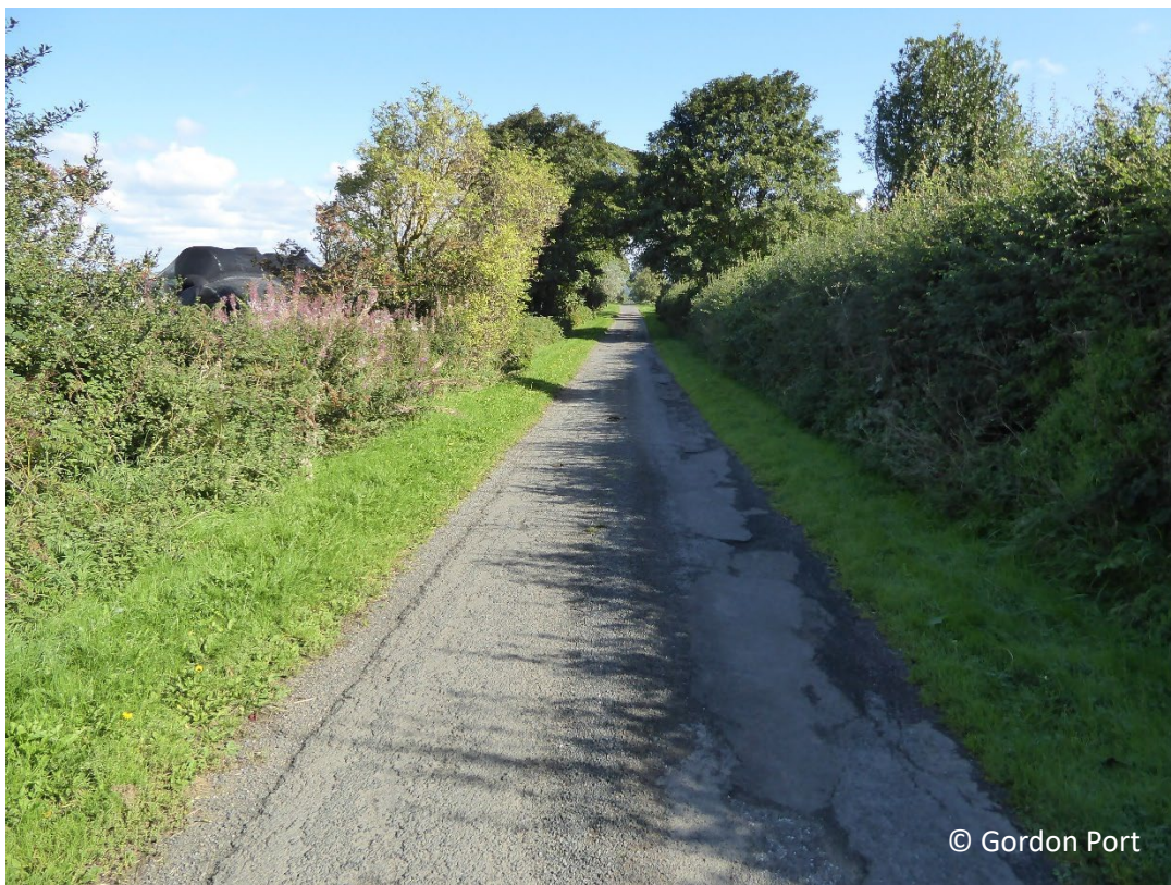
P3 Looking northeast along road. September 2023
